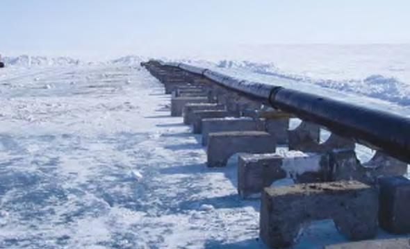
Installing concrete anchors on insulated HDPE intake pipeline – anchors secured with stainless steel bolts.
