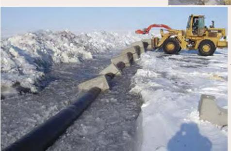
Installation of insulated and anchored HDPE using strategically placed heavy equipment – ice platform used for intake installation.
