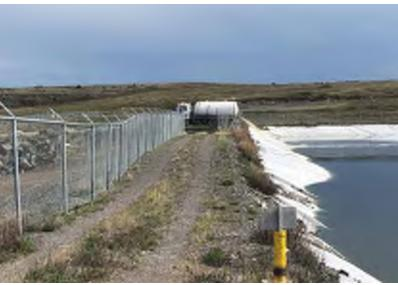
An extensive field program was initiated in 2021 to investigate the potential causes of the lagoon issues and form the basis for remedial work. Site reconnaissance was completed focusing on settlement and drainage issues (See subsidence in top of fence line). Topographic elevations were recorded to help quantify the historical subsidence any continuing subsidence in the berms.
