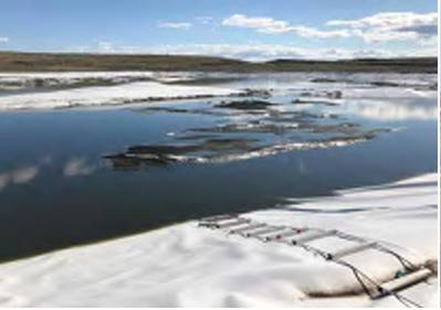
The Kugluktuk lagoon was constructed in 2008 consisting of a 240-metre and 200-metre cell lined with an HDPE liner. A major issue o ccurred with the formation of "whales" in the liner, seepage from the base of the lagoon and subsidence in the top of the lagoon.
