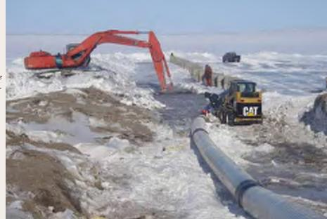
Preparation for intake installation with removal of ice and excavation of the lake bottom.
